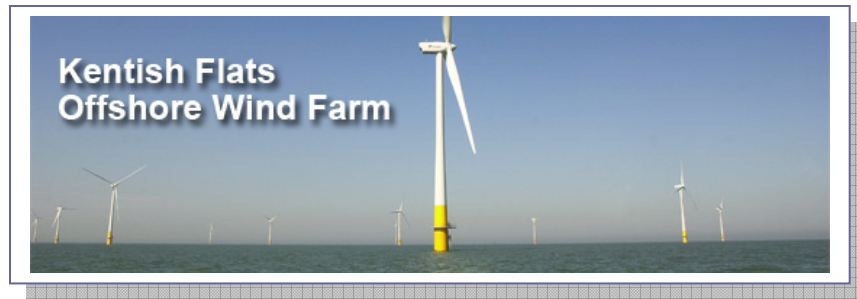
Figure 11: A commercial offshore wind farm in the UK (43)
